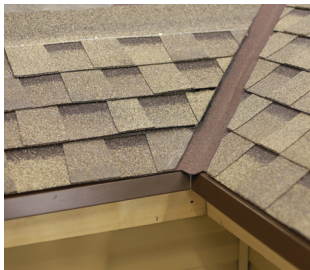
Valley installed by open method.
